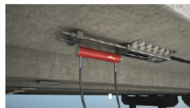
fixing jack and anchor bolt
