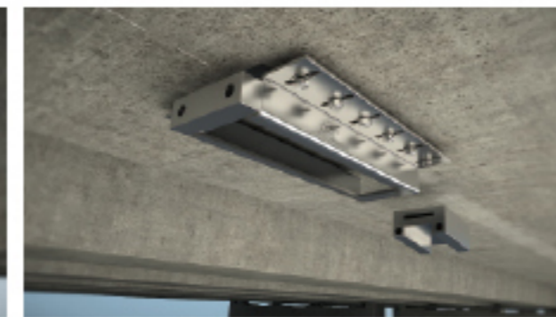
installing anchor block
