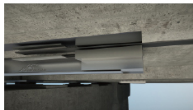
fixing carbon fiber laminate
