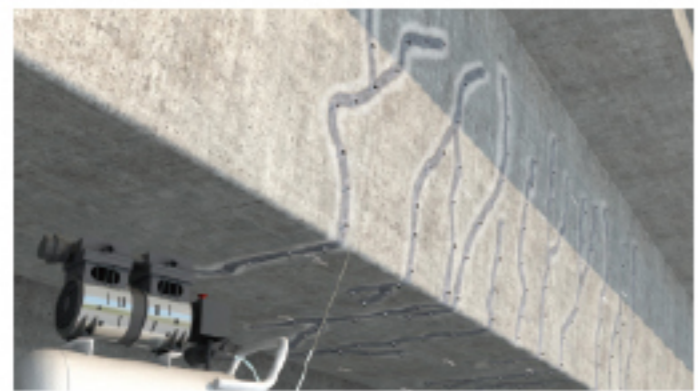
sealing inspection
