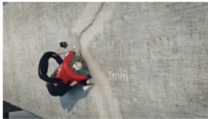
crack treatment
