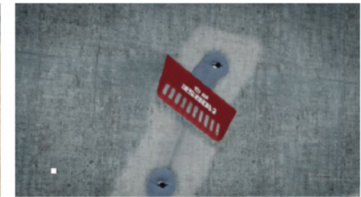
sealing crack
